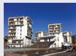
SOCIAL HOUSING CANTIERE VIA CENNI MILANO
