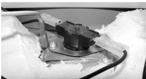
Fig. 23: Safety thermostat reset button
