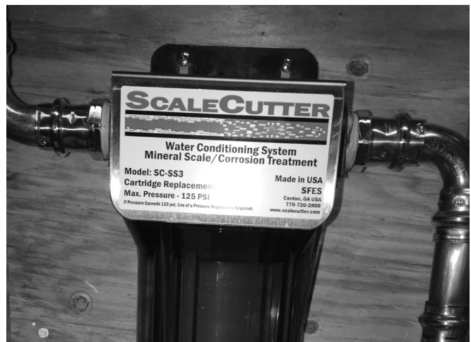
Figure 4.5: ScaleCutter® Water Treatment System for Domestic Water Plate Heat Exchanger Protection.
