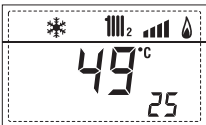
26. Safety thermostat with MIX 2 ZONE board (input S1), respectively ON and OFF
