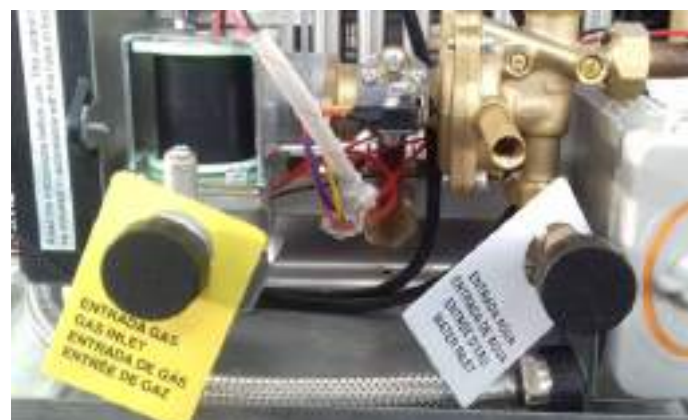
fig. 8 - Connection cards
