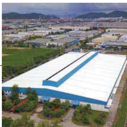
Nuovo Fujitsu General Co., Ltd. (Tailandia) FACTORY-2
