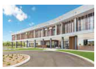
Fujitsu General (Aust.) Pty Ltd. (Australia)
