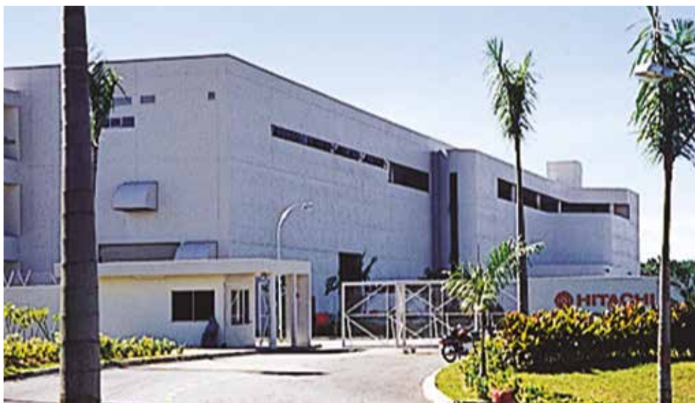
Hitachi Air Conditioning Products (M) - Stabilimento HAPM - Kuala Lumpur, Malesia
