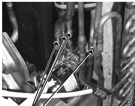
Welded parts of 4-way valve
