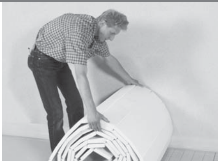
Posare i pannelli Tacker.
